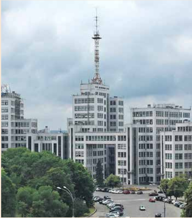
Derzhprom (State Industry House), Kharkiv, 2018. Built in 1928, it is the oldest skyscraper complex in Europe.
